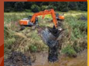
Breaching the old bank on the River Tamar. Photo courtesy Steve Haywood
